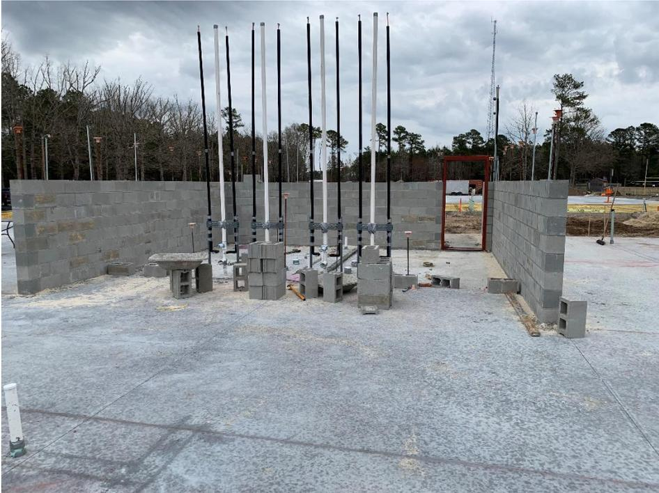
Supply water, hot and cold, comes from the overhead to alleviate some of the problems we have experienced in the past with pipes leaking under concrete. The wall on the right was one course of block tall on Wednesday. The seven course limit per day on laying blocks is to give the mortar time to harden thereby not allowing the wall to tilt or even fall over.
