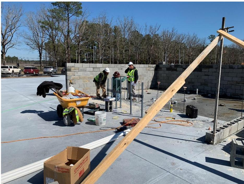
This picture of the group restroom in the eighth grade wing. This picture was taken on Wednesday. The boards are braces for the corner post the masons use to pull strings to lay the blocks to keeping the wall straight.
