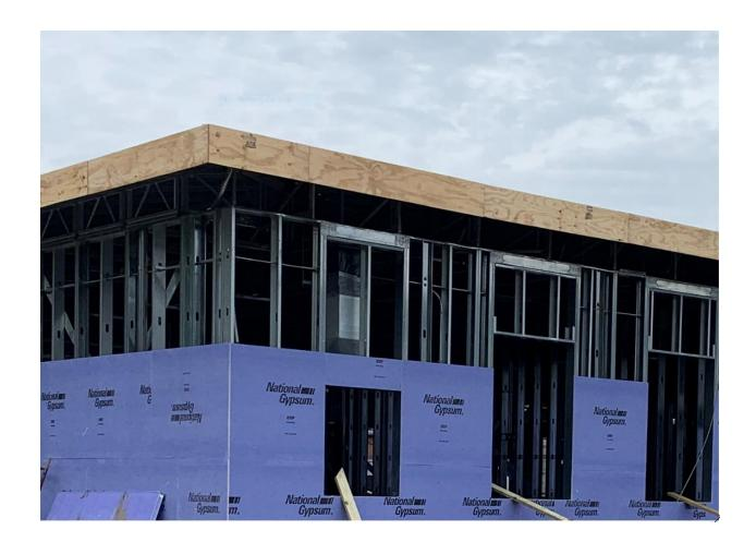
Half inch plywood has been added outside the 2 X 6 perimeter. The plywood covers the 2 X 6 pad and comes down to the bottom of the face across the end of the trusses to serve as an attach point for the roof edge covering. The 6" thick insulation will lay inside the 2 X 6 perimeter.
