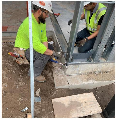
The next photo is a closeup of the above picture. Notice the hatchet used as a pry bar to make room for the tray slipping in from the west. Notice both workmen are wearing safety glasses and both are wearing cut resistant gloves. Not all work sites display this regard for safety.
