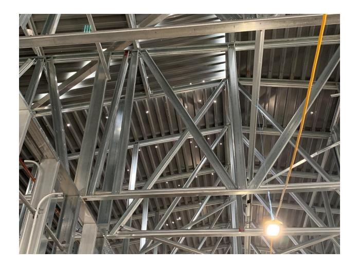
After talking with Brian Plyler I learned the holes were made when lanyards were secured for workmen on the roof. Some holes were possibly made when workmen were attaching the sheets and missed the truss location. All this will be covered with 6" thick Styrofoam insulation next week then more weatherproofing material and finally the standing seam roof.
